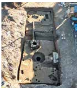
A photo of excavational investigation
